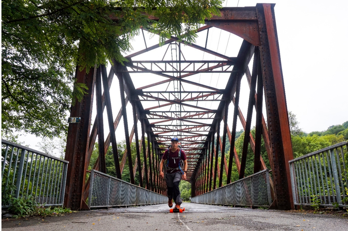
Figure 18 - Bike path bridge
