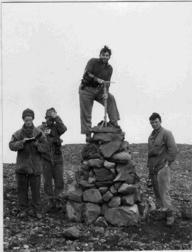
Fig. 23: Typical cairn as built during the Thrandarjokull ice cap survey
