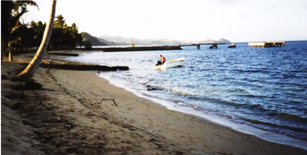
The pier at Sawana is broken
