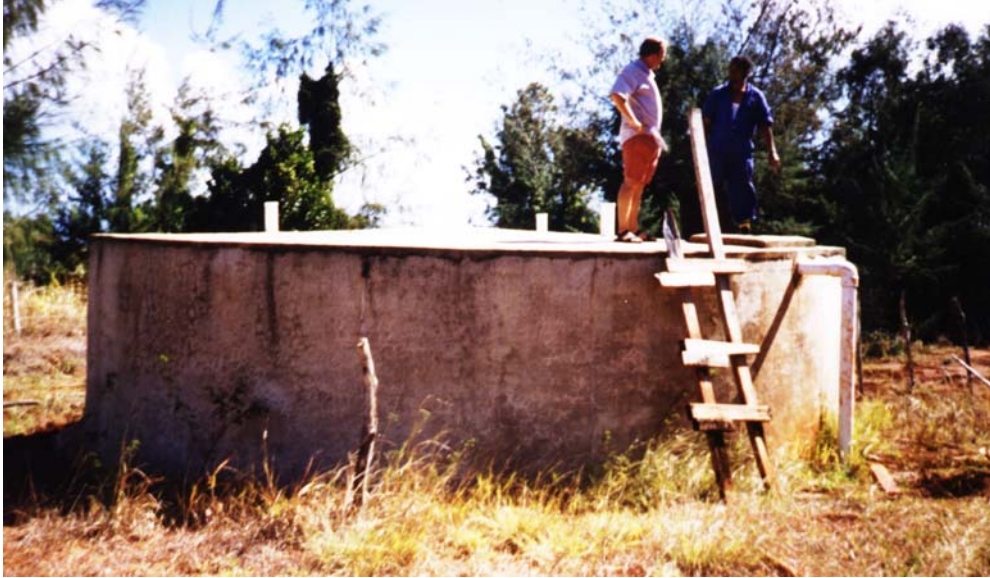
This 20,000-litre tank, near to Malaka, was generally filled at night – but had no stop valve and was prone to overflow. It represents the islands main reserve tank.
